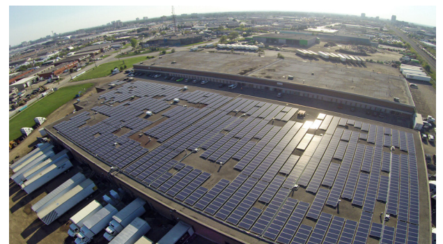
600 kW DC FIT 2 Project located in Brampton, Ontario, completed in July 2015.
