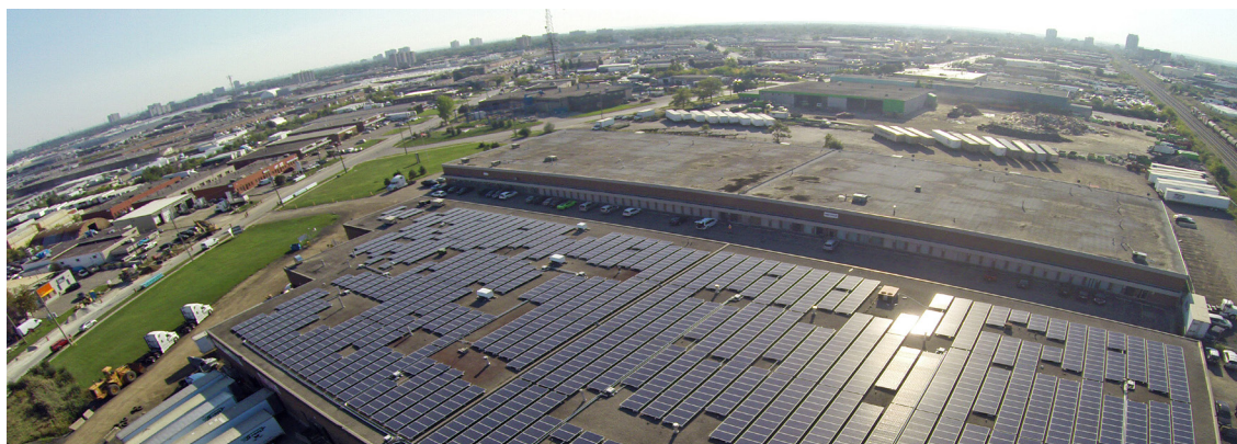
600 kW DC FIT 2 Project located in Brampton, Ontario.
