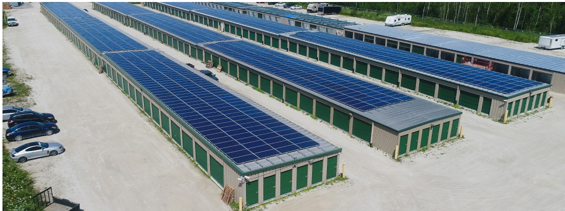
400 kW DC FIT 3.1 Rooftop Project located in Wasaga Beach, Ontario.
