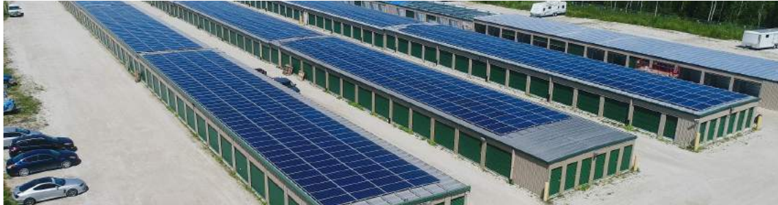
400 kW DC FIT 3.1 Rooftop Project located in Wasaga Beach, Ontario.
