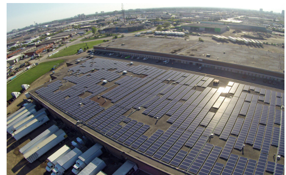
600 kW DC FIT 2 Project located in Brampton, Ontario.
