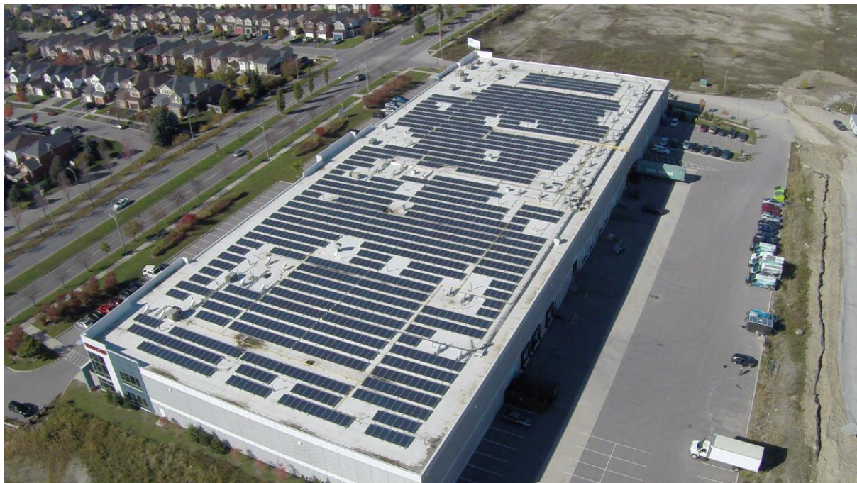
Shot of one of the 2012 LP's FIT 2 600 kW DC projects, brought online in July 2015.
